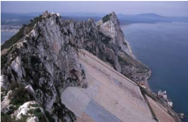
Water catchment sheets covering the East Side sand slopes 1989 (above)
