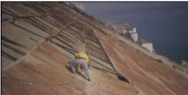
Water catchment sheets covering the East Side sand slopes 1989 (above)
