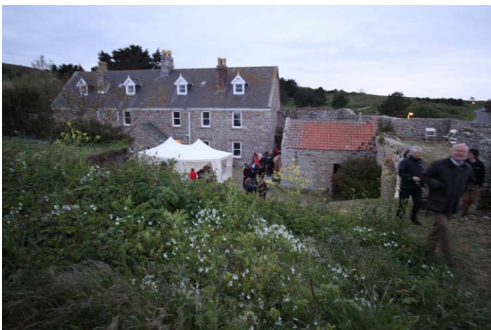
The Nunnery on Alderney, where Bird Observatory volunteers are housed. The building is a historically important structure, with fortifications from Roman, Tudor, Victorian and World War2 periods. (The marquee is for an evening event.) Photo: Dr Mike Pienkowski
