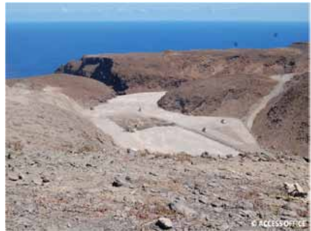
St Helena Airport Dry Gut infilling: 7.6 million cubic metres of rock dumped and compacted to maximum height of 120m
