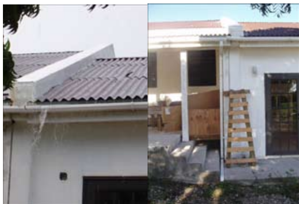
Roof and gutter – both had major leaks. The gutter was rebuilt, and the roof leaks plugged from inside and out. Also showing the home made ladder; the proper one had gone missing but re-appeared late in our stay.
