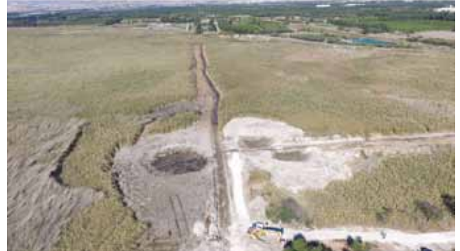
Habitat creation work at Akrotiri. Photo: Akrotiri Marsh Project.
